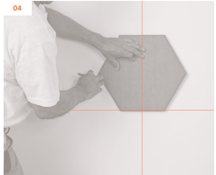
Match the center point of the panel with the center point of the wall, and apply the panel to the wall.
