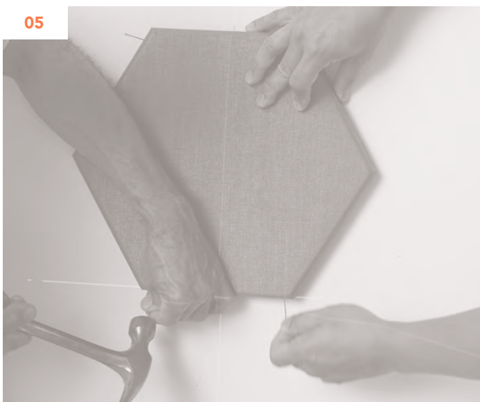
Push a pin through the side of the panel and into the wall. This holds the panel up until the Quick Grab Formula dries. We recommend pinning the entire first row.
