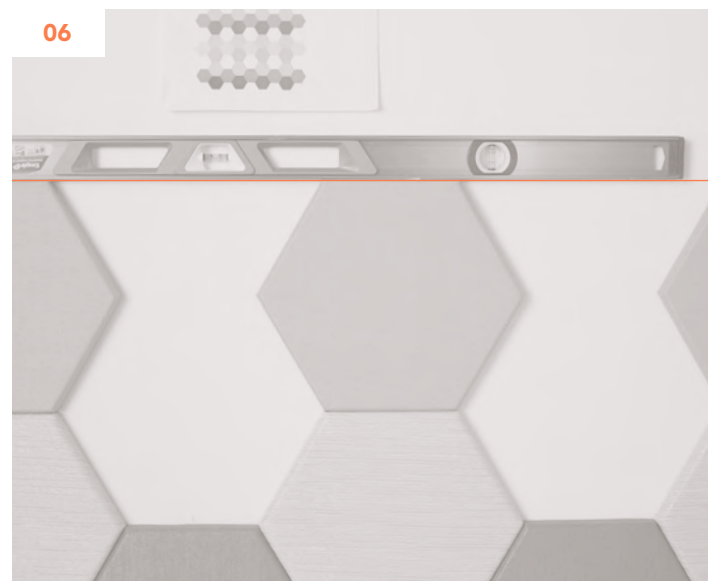
As you install additional panels, interlock each panel to minimize gaps. Once multiple panels are installed, make sure they are level and square using a level or laser. Finally, clip the tops of the pins once installation is complete and secure.
