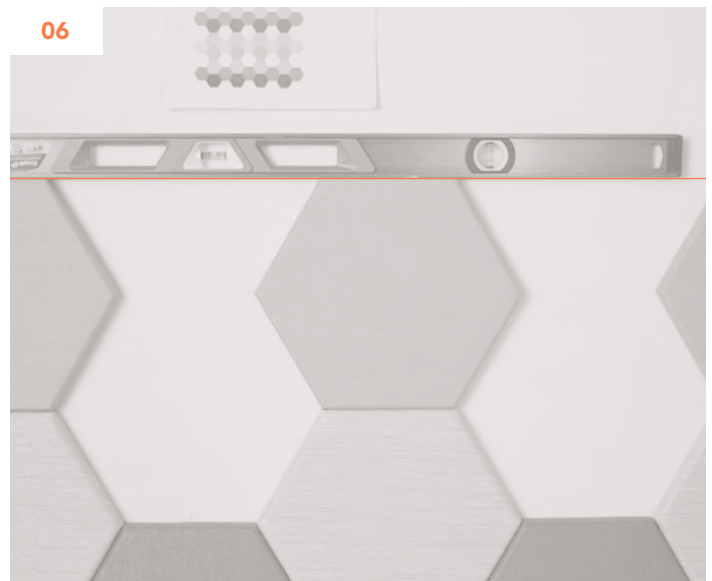
06 Once multiple panels are installed, make sure they are level and square using a level or laser.
