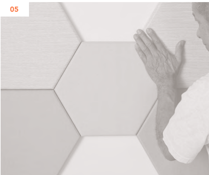
05 Apply pressure to the sides of the panel to make sure the panel is secure. As you install additional panels, interlock each panel to minimize gaps.
